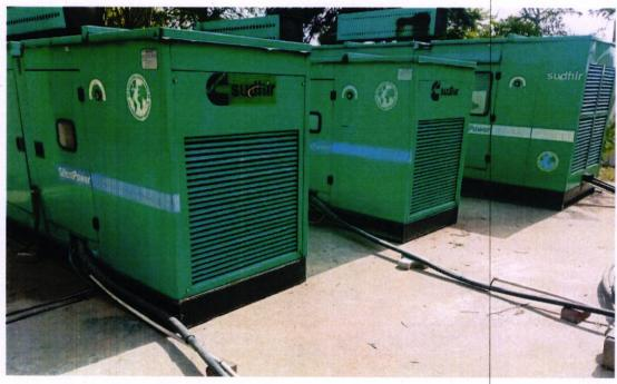
**Observation and Suggestions:**- As per the trial taken during the energy audit the percentage loading of DG set is 66.28% which is ok and specific energy consumption of DG Sets 3.49 KWH/Litre which is satisfactory because as per manufacturer recommendation, best practices for SEC in DG sets range from 3.0 to 3.5 kWh/litre and above.
